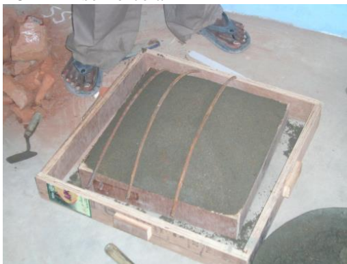
Fig.1.Construction of funicular Shell
